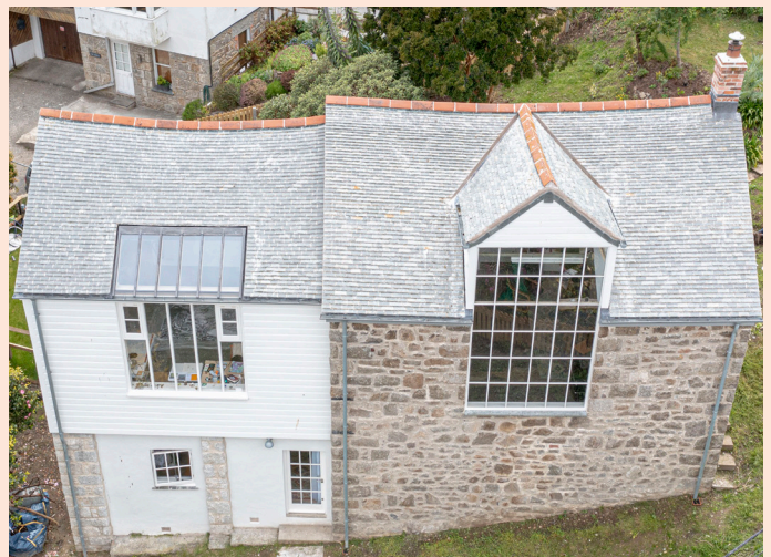
North Elevation in May 2021 after renovation
